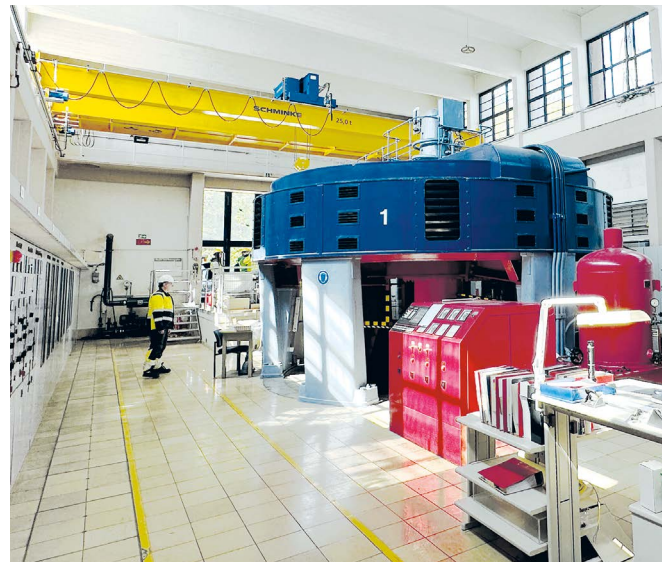
Maschinenhaus in Rothenfels
