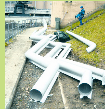
Zigzag tube for downstream fish migration in Rothenfels.
