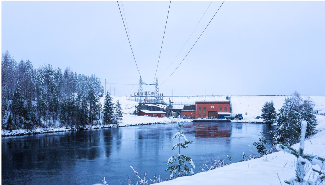
A Uniper Hydro plant in Sweden
