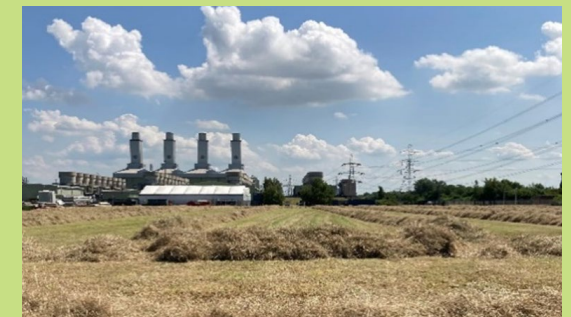
Connahs Quay Power Plant in the United Kingdom
